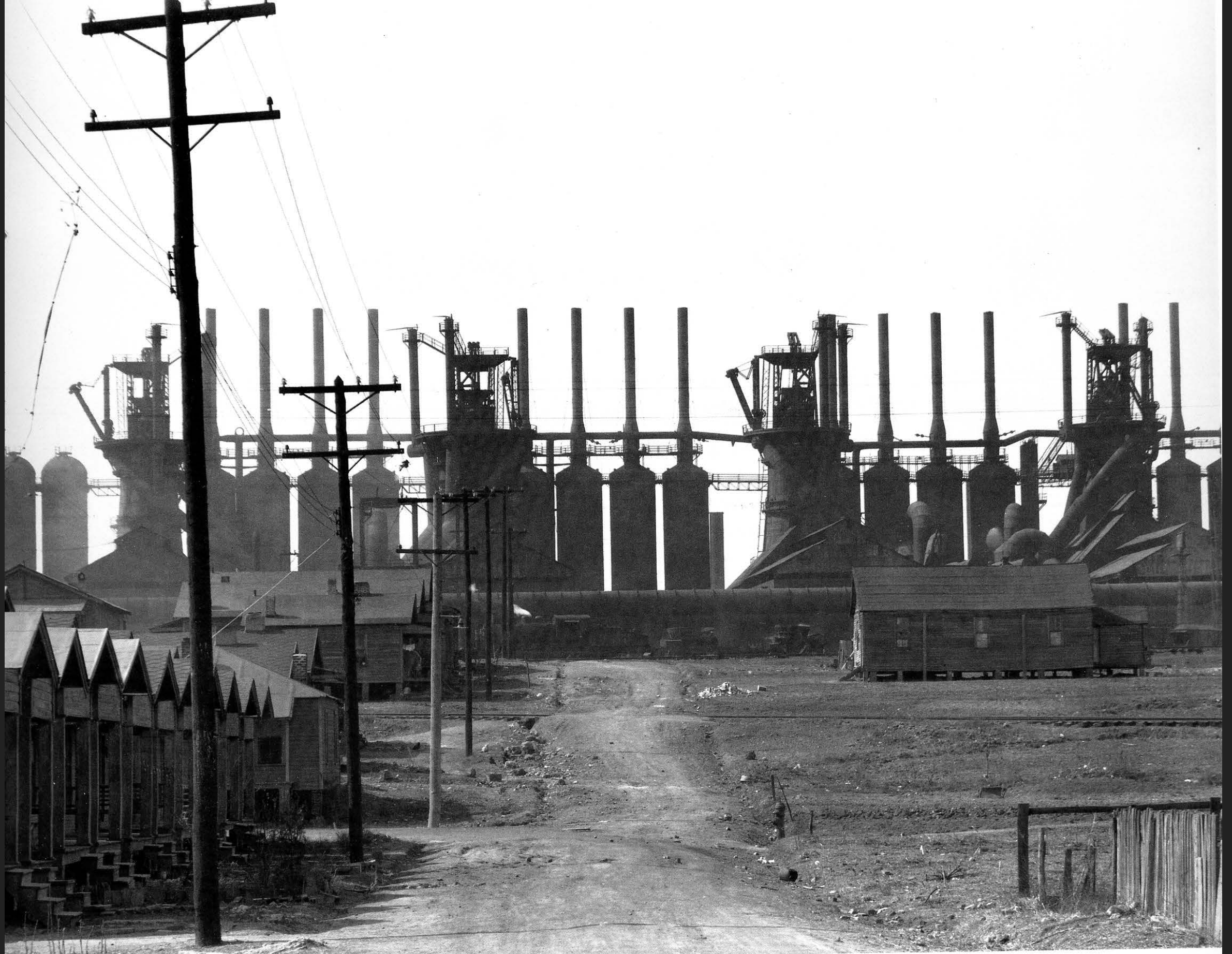
STEEL MILL & COMPANY HOUSES
